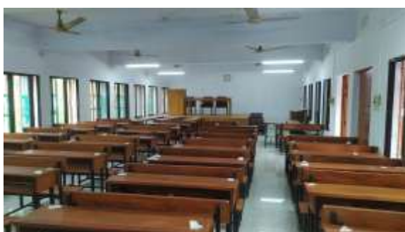
Refurbished Classroom cum auditorium.
